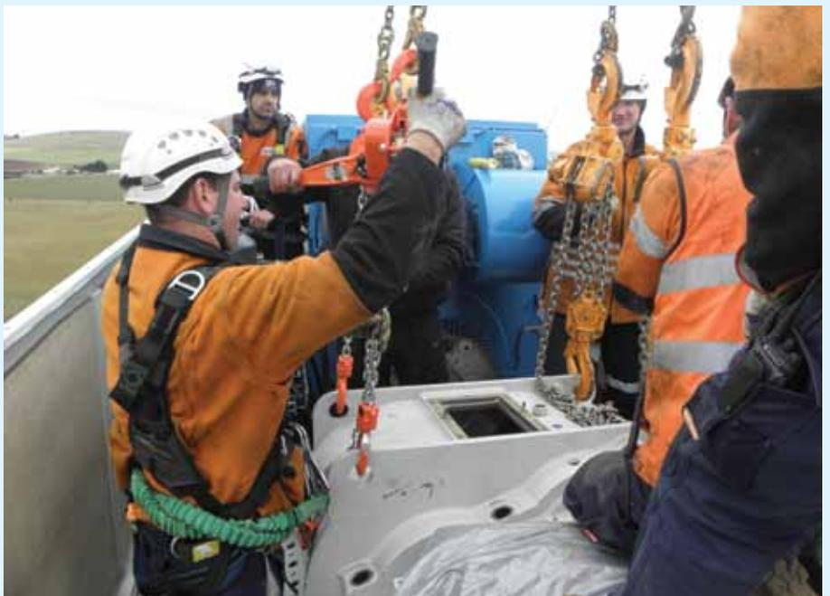
*The top of the nacelle was temporarily removed for this gear box change on turbine 3A2*
